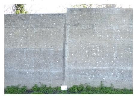
Figure 3 – Section of Wall in in-situ mass concrete
