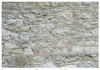
Representative section illustrating loss of ribbon-pointing
